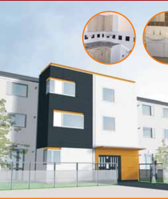
above, Beardsfield improvements; insets, Smiths Point kitchen and bathroom refurbishments
